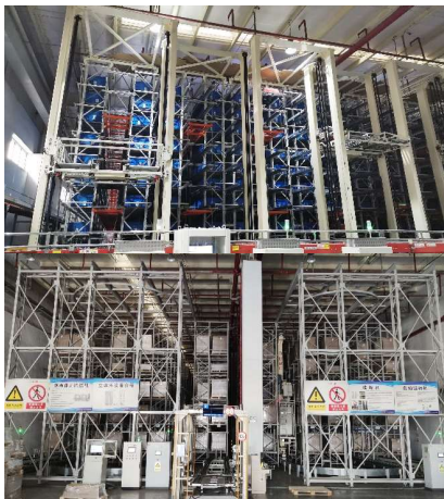
HEFEI 2017 FG WAREHOUSE
